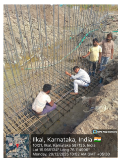
Joint inspection of construction of retaining wall at ilkal under the supervision of municipality ilkal by Prof. S. A. Kambli
